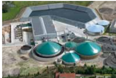
Aerial view of the biometanisation plant in Ardoorie, Belgium
