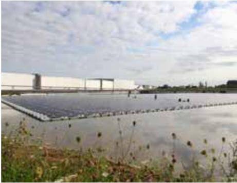
A unit of floating solar panels has been installed in the water basin at the Ardo site in Geer. Spanning an area of one hectare, the floating solar panels are a first in Belgium and will generate at least 1,000MWh (megawatt-hours) in 2018. This equates to the electric consumption of 300 households (the equivalent of the number of employees at Geer)! This will allow Ardo Geer to increase its self-generated renewable energy to 30%.
